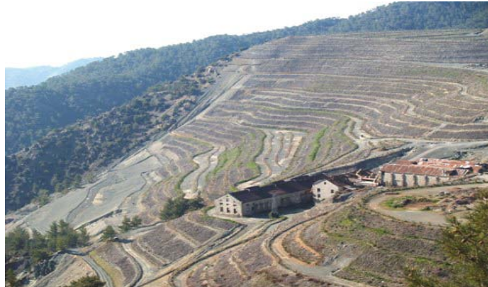
A picture showing terraces after reshaping and restoration
